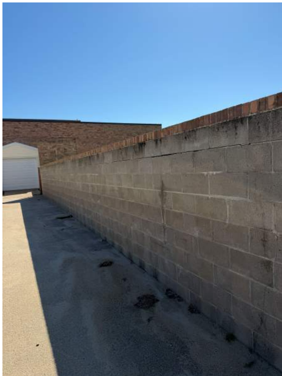
PHOTO 4 - LOADING DOCK RETAINING WALL
