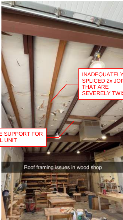
PHOTO 10 - CTE ROOF STRUCTURE
